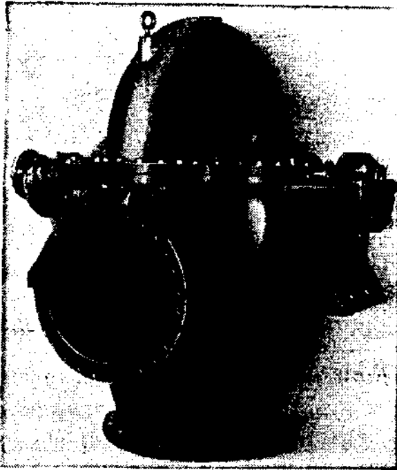
FIG. 2-7. View of double-suction pump with bottom suction.
